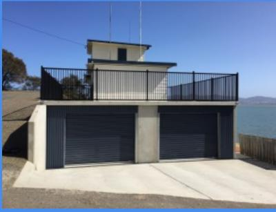
On Wednesday 27th the framing and roller doors were fitted and Feb 2 the doors were fitted and now we have the final cladding and windows installed.
