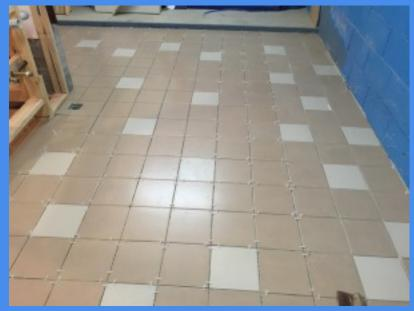
After a significant delay considerable progress has been made on the change rooms upgrade with floor tiles being laid, the water proofing of the shower bays and new partitions being constructed.
